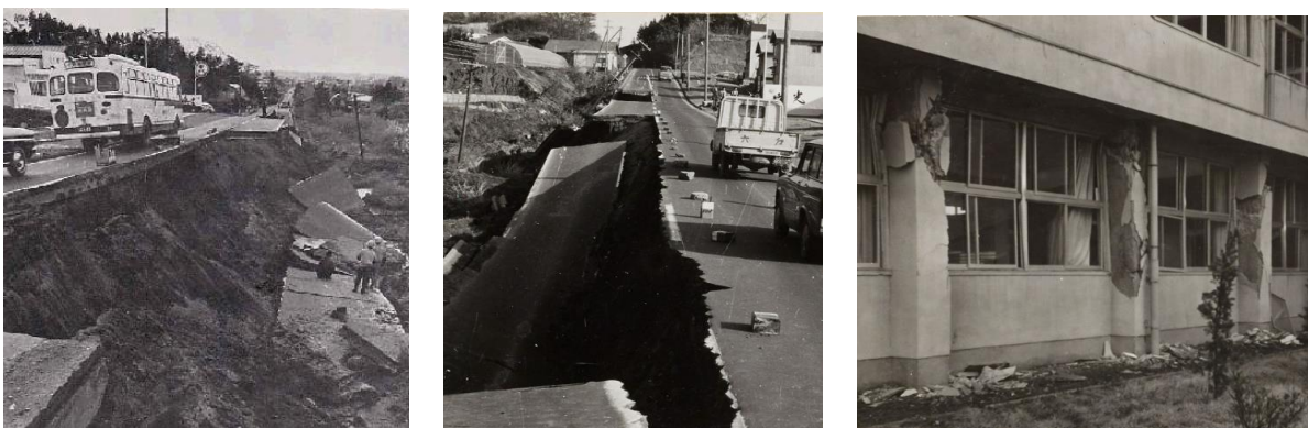
Figure 12. Damage by the 1968 Tokachi offshore Earthquake (Hachinohe City)
