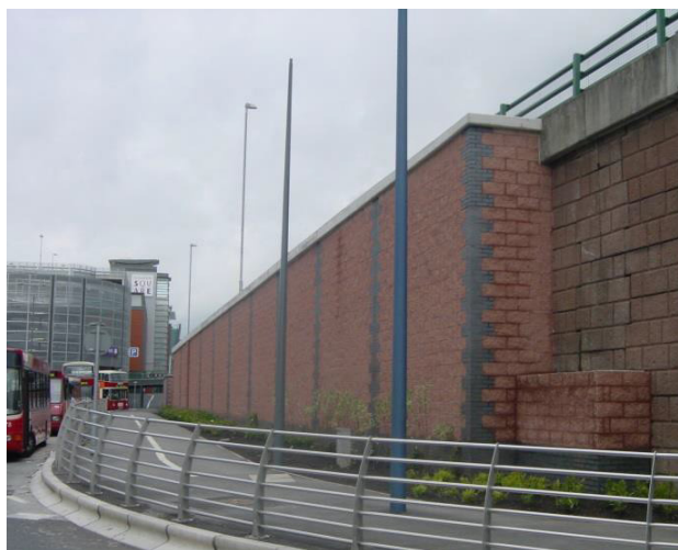
Figure 9: Installation & Excavation Retaining Wall (Completion)
