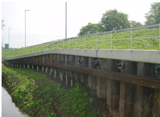
Figure 7: Installation & Filling Retaining Wall (Completion)
