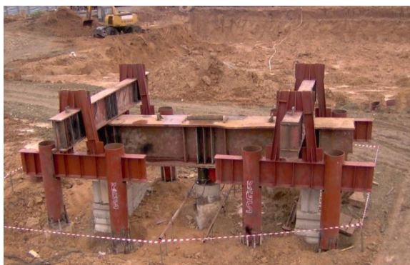
Figure 1. Field static load test of CFA1 on construction site (Building 3)
