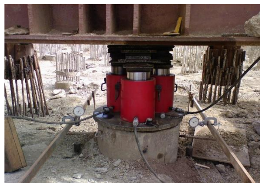
Figure 2. Field static load test of Casing2 on construction site (Building 5)
