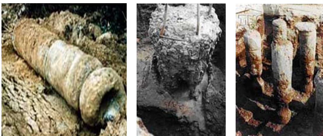
Figure 6. Examples of defective piles
