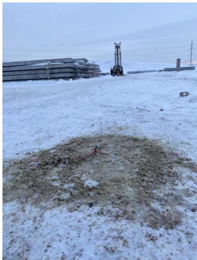
Figure 10. Spreading the antifreeze reagent on top of snow Figure 11. The pile installation on thawe
