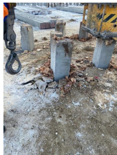
Figure 10. Spreading the antifreeze reagent on top of snow Figure 11. The pile installation on thawe
