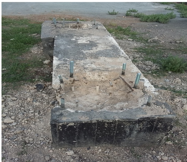
Figure 3. General view of the pile grillage
