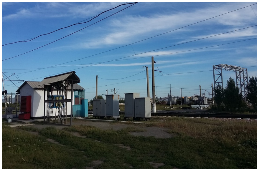
Figure 1. General view of the construction site
