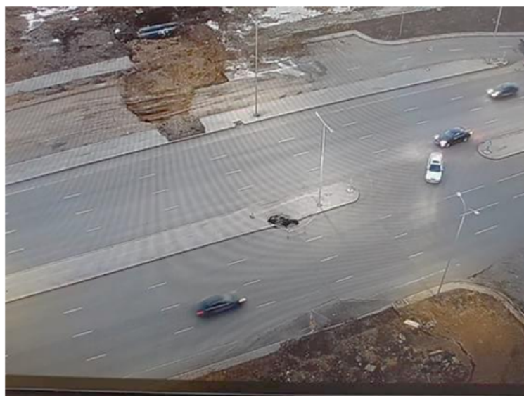
FIGURE 1 – Frost-thawing problem related hazardous situation in road on ChingizAytmatov str. in Astana
