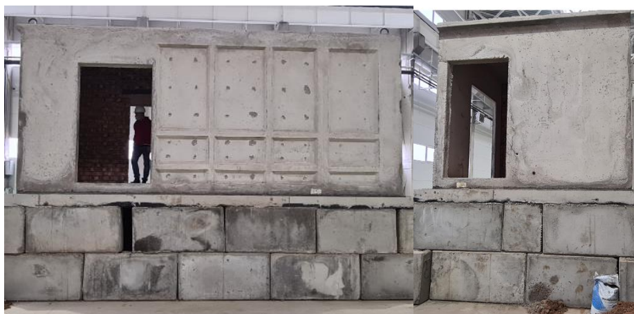
Figure 2. General view of the volumetric block on the pedestal
