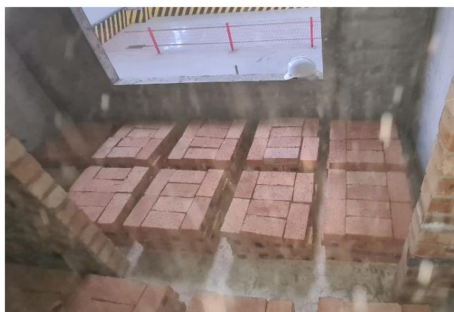
Figure 4. View of loading the floor slab with bricks
