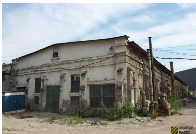
Figure 1. The Almaty Electrotechnical Plant (before adaptation)
