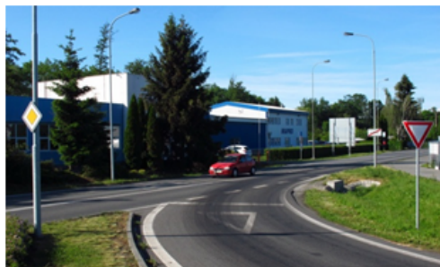
FIGURE 17 – Bypass with dead angle on turbo-roundabout in Olomouc (road I / 35, Czech Republic).
