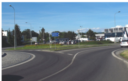
FIGURE 6 – Exit with two exit lanes (one lane offers choice for direction) on turbo-roundabout in Olomouc (road I / 35, Czech Republic).
