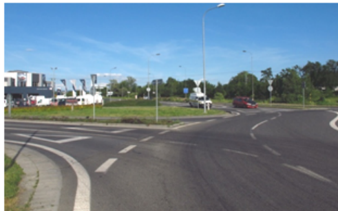
FIGURE 5 – Yield to two lanes during entering turbo-roundabout in Olomouc (road I / 35, Czech Republic).
