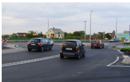
FIGURE 20 – Lane dividers used on turbo-roundabout in Erd (roads no. 6 and 7, Hungary).
