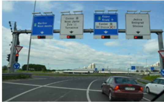
FIGURE 9 – Direction traffic sign for each traffic lane separately placed above entry lane on turbo-roundabout in Slovenia [2].
