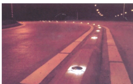
FIGURE 21 – Lane dividers with lights used on turbo-roundabout in the Netherlands [7].
