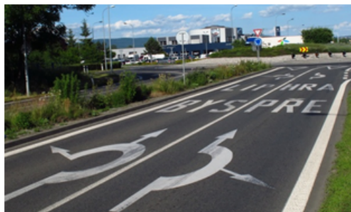
FIGURE 16 – Writings on the traffic lanes before entering turbo-roundabout in Olomouc (road I / 35, Czech Republic).
