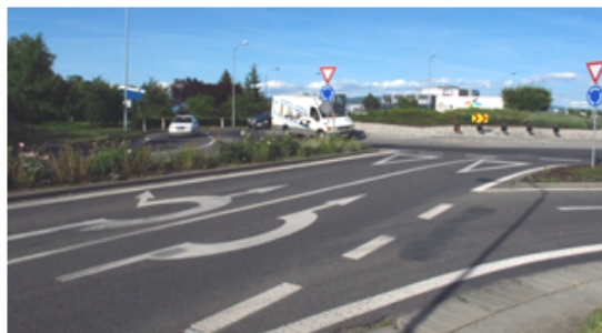
FIGURE 11 – Road markings with a symbol of a roundabout before entering turbo-roundabout in Olomouc (road I / 35, Czech Republic).
