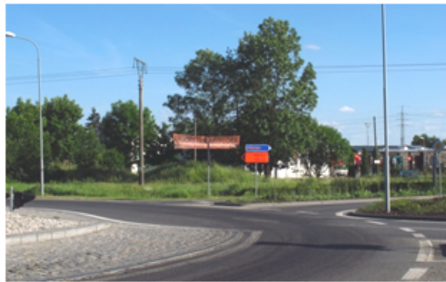
FIGURE 4 – The nested spiral lane on entry of turbo-roundabout in Olomouc (road I / 35, Czech Republic).
