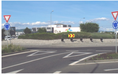
FIGURE 3 – The nested spiral lane on entry of turbo-roundabout in Olomouc (road I / 35, Czech Republic).
