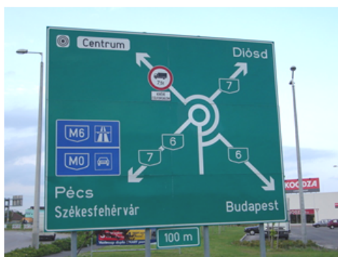
FIGURE 7 – One direction traffic sign showing all directions on turbo-roundabout in Erd (roads no. 6 and 7, Hungary).
