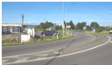
FIGURE 18 – Safe and correct bypass on turbo-roundabout in Olomouc (roads I / 55 and II / 570, Czech Republic).
