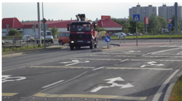
FIGURE 12 – Road markings with a symbol of a roundabout before entering turbo-roundabout in Erd (roads no. 6 and 7, Hungary).
