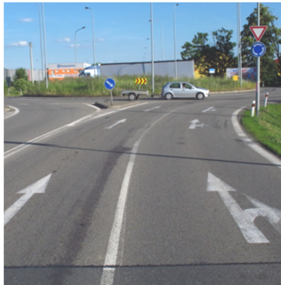
FIGURE 15 – Normal arrows used (as road marking) with traffic sign “Roundabout” before entering turbo-roundabout in Olomouc (roads I / 55 and II / 570, Czech Republic).
