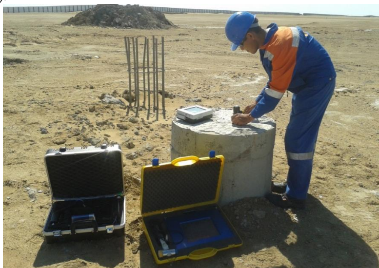
Figure 5. Performing pile integrity test
