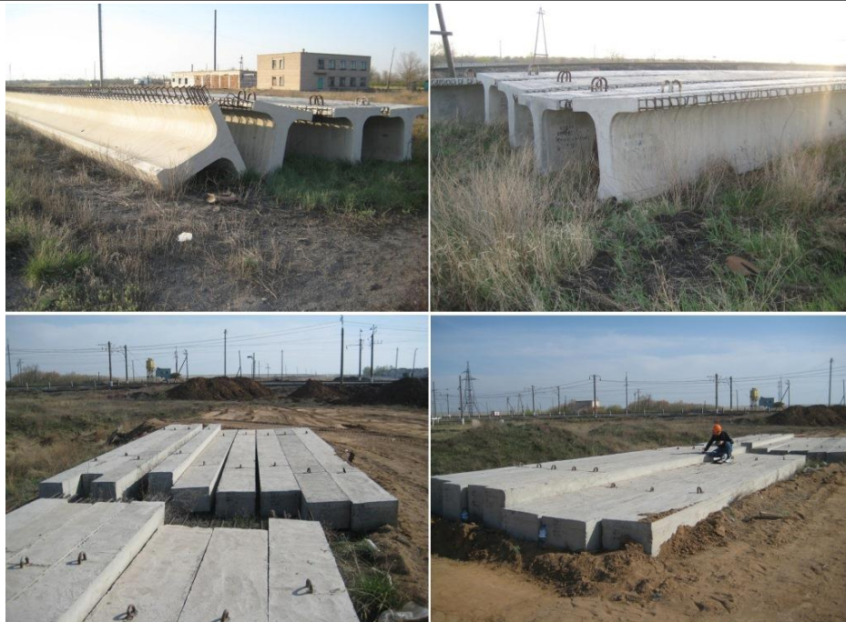
Figure 3. Supports and beams
