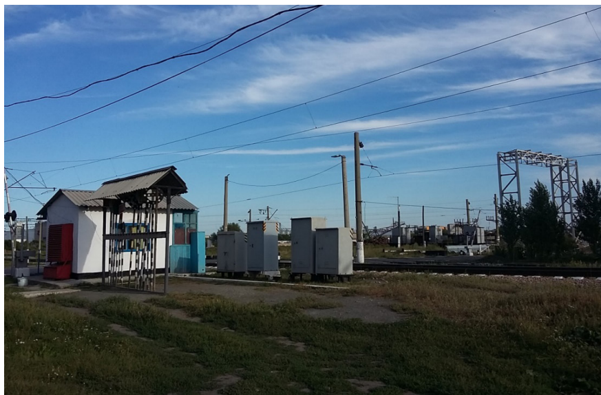
Figure 1. General view of the construction site
