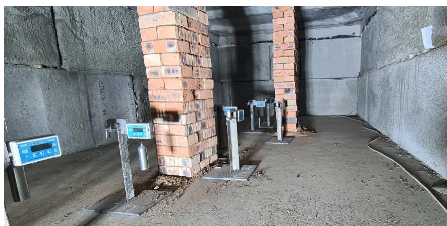
Figure 6. Fragment of a concrete pedestal
