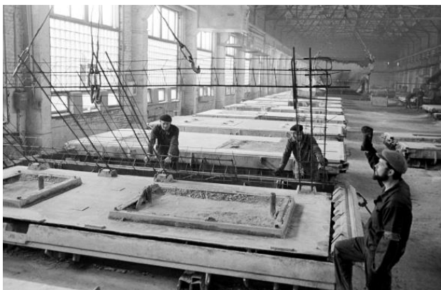
Figure 7. Almaty House-Building Plant (before adaptation)
