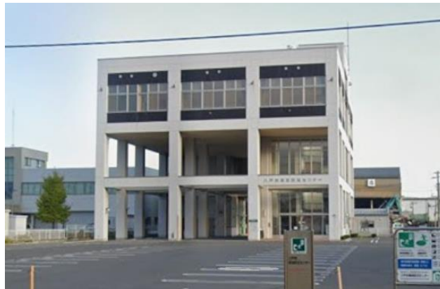
Figure 18 Tsunami Disaster Prevention Center in Hachinohe Constructed for tsunami evacuation purposes in a low-lying area with no nearby elevated ground.
