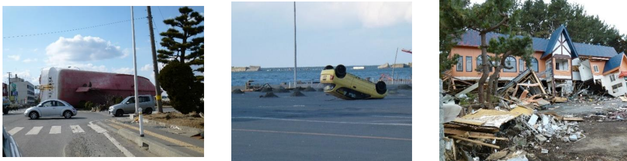
Figure 14. Damage by the 2011 Tohoku Region Pacific Ocean offshore Earthquake and Tsunami
