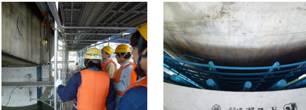
Figure 15 Seismic reinforcement of bridge piers by PC panels (2012, Yanagibashi Bridge, Hachinohe City)
