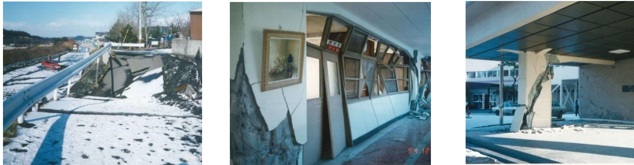
Figure 13. Damage by the 1994 Sanriku far offshore Earthquake (Hachinohe City) Left Slope collapse (from Morioka Meteorological Observatory website), Center) Damage to buildings (ibid.) Right Damage to buildings
